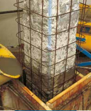
Gieten in bekisting
